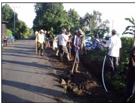
The local community laying pipes
