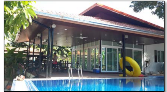
The first house built by the young men
